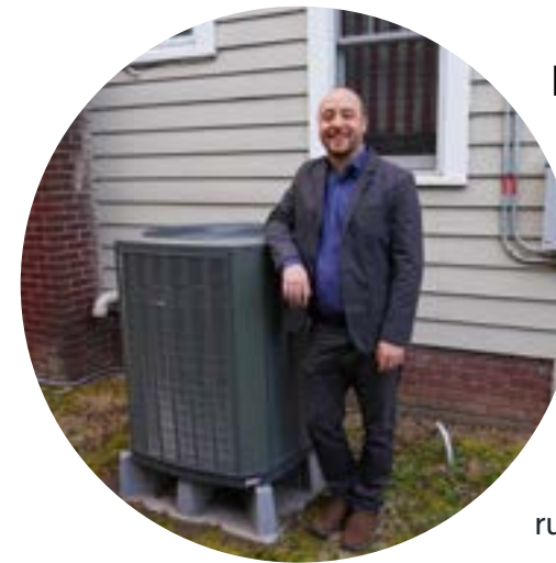
KIRCHER NEXT TO HEAT PUMP OUTSIDE PURDUE’S DC NANOGRIID HOUSE (PHOTO: PURDUE UNIVERSITY/JARED PIKE)
